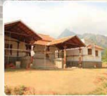
VILLA CONSTRUCTION AT FULL SWING BY PURCHASER
